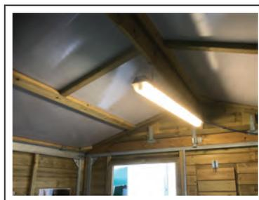
The suspended fluorescent tube and insulated roof. Note the position of the rear door.
