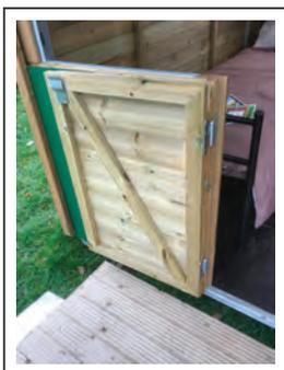
The Barn Door in the open position. The doors can also be lifted off their hinges and removed completely.
